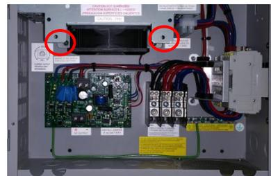
**Step 4.** Position the new module in the Clipper chassis with the terminal block toward the middle of the Clipper and slide the mounting tabs into position. Secure the module with the screws removed in **Step 3**.
