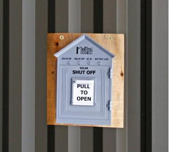
On an uneven surface it is recommended to mount a flat panel to the wall and mount the Birdhouse on the flat panel.
