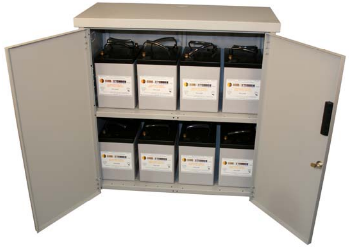
MNBE-B enclosure with eight Concorde PVX-2240T's installed
