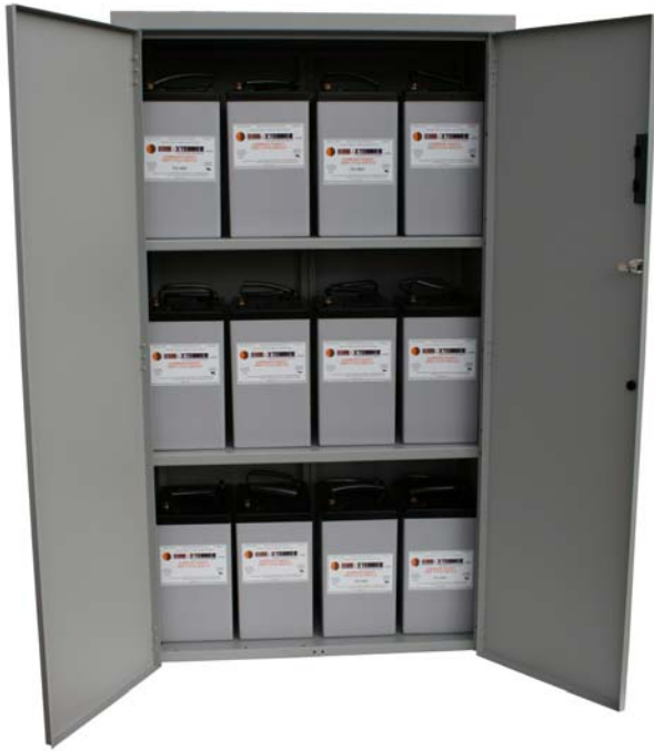
MNBE-C enclosure with twelve Concorde PVX-3050T's installed
