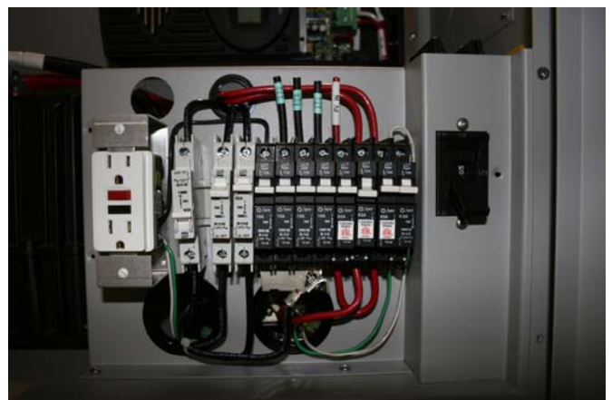
Breakers with cover removed. Note the PV and DC-GFP breakers on this system.
