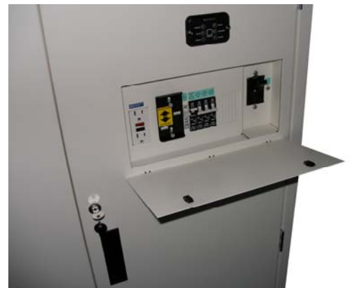
Transfer switches and circuit breakers are concealed under a hinged door
