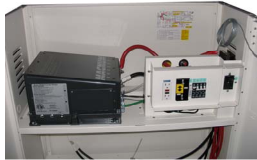
Magnum modified inverter installed in the “C” system enclosure.
