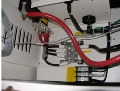
Internal wiring showing the optional plus and minus busbars.
