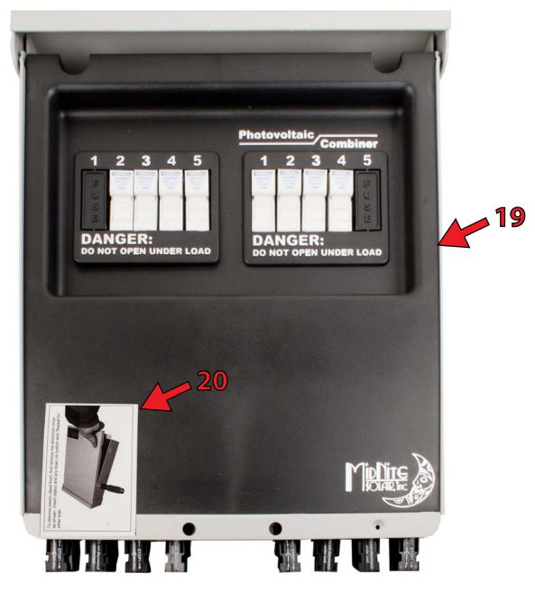
Step 19. Attach the deadfront #5-032-1, placing the bottom end tabs into holes in the chassis and snapping in the top.
