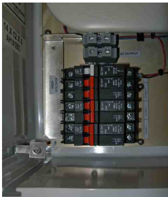
Large busbar re-installed
