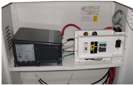
MNBE-C-250 with Magnum inverter installed
