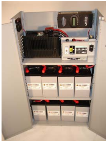
MNBE-C-175 built for battery back up grid tie by SunWize Technologies
