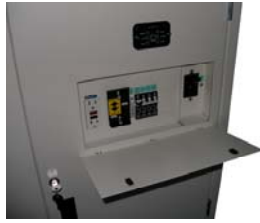
Flip down door hides a compliment of breakers
