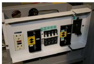
**Grid/Gen version has an AC input transfer switch. This allows the customer to simply plug in a portable generator to re-charge batteries during a prolonged power outage. A 50 amp breaker is used on the utility position and a 15 amp is used on the generator position.**
