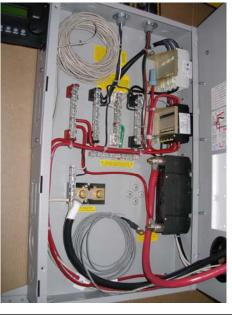
Magnum all wired up with lightning arrestors, charge control disconnects, DC-GFP and remote display ready for transport to the job site. Note that this picture is of a previous version prior to the addition of the PV plus input busbar.
