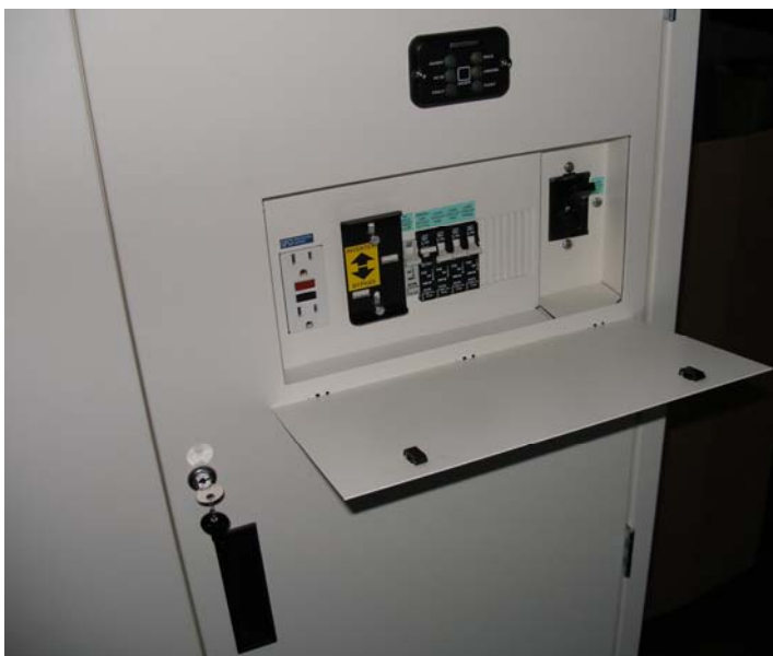
This photo shows the breaker cover installed.
