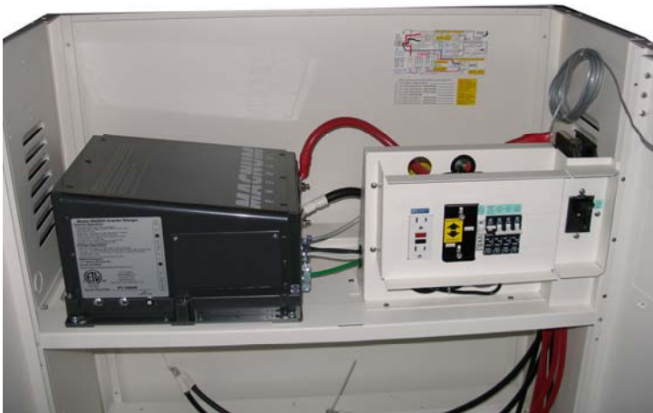
This photo shows the breaker cover installed.
