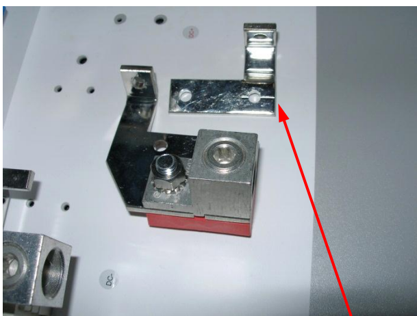
Remove two bolts holding small busbar. Remove small busbar from PV positive lug
