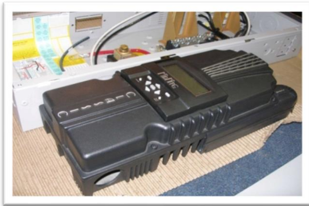
Figure 4 – Classic mounted to E-Panel
